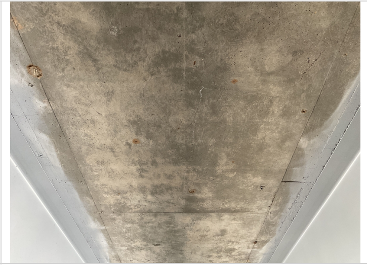
Efflorescence in underside of deck
