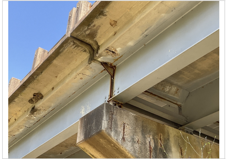
Span 1 corrosion
