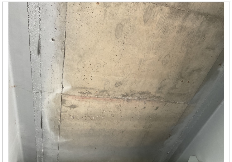
Cracking on underside of deck
