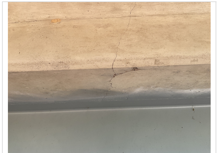
Cracking on underside of deck
