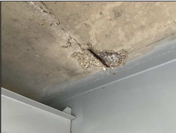
03/2022... end span spall
