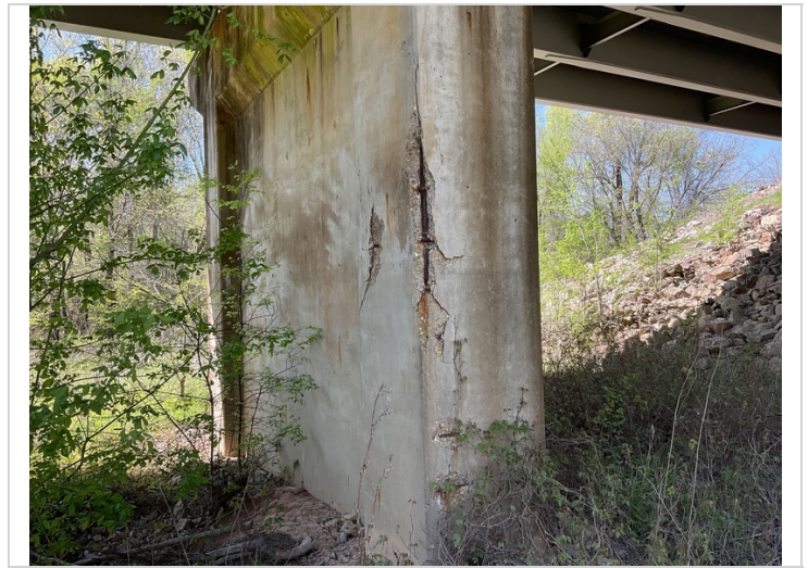
Bent 3 column 2 CS3 rebar exposed
