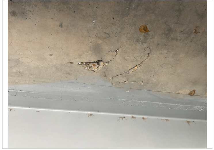
Delaminations on underside of deck
