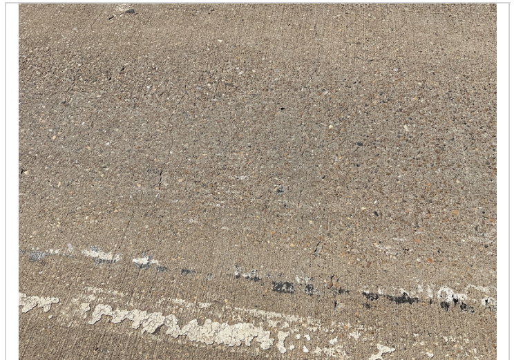
Sealable deck cracking
