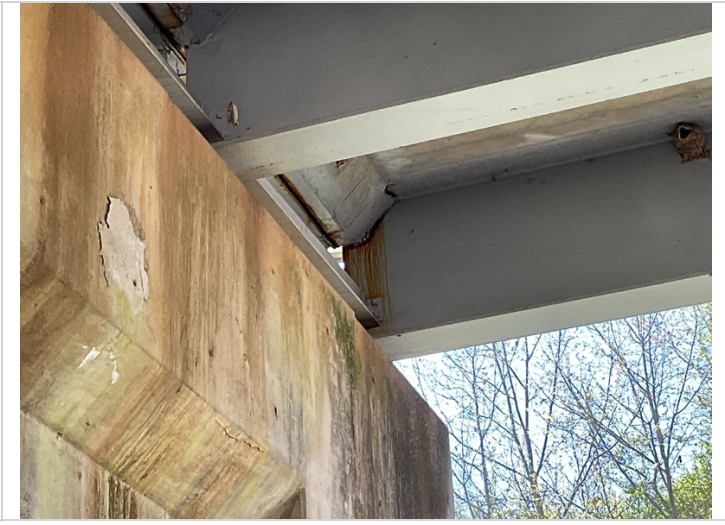
Beam end corrosion bent 3
