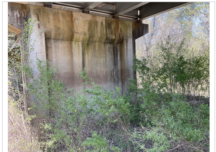
Pier wall at bent 2 rebar exposed
