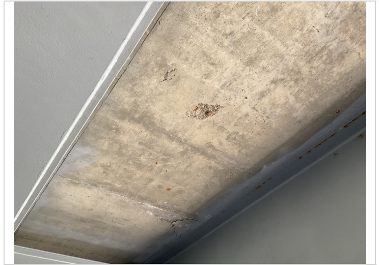
Spalls on underside of deck
