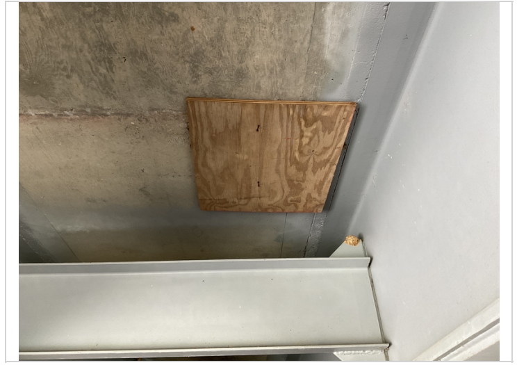
Patched area underside of deck
