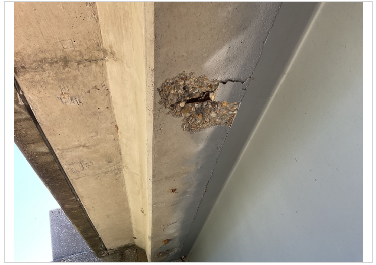
Span 1 underside of deck Rt side rebar exposed
