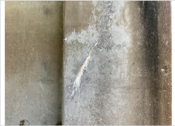
Bent 2 column 1 efflorescence
