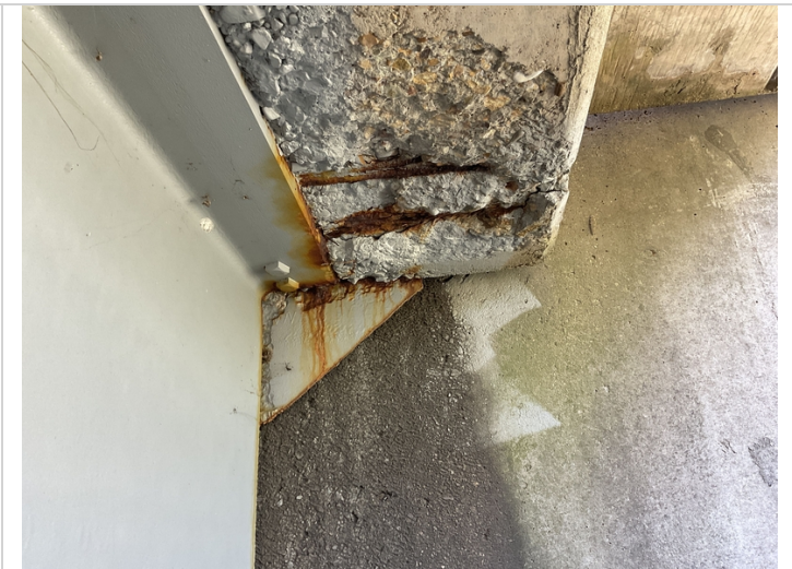
Exposed rebar span 3 RT side
