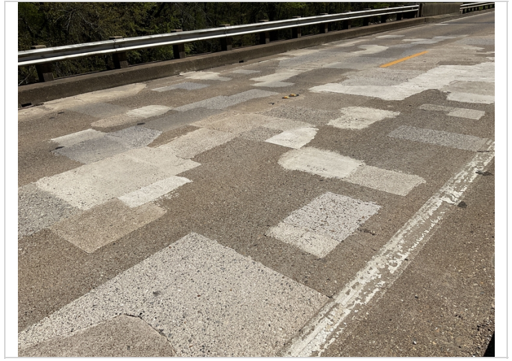
Span 1 patched area
