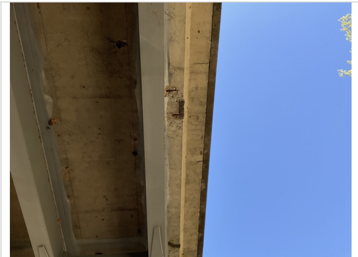
Exposed rebar on overhangs.
