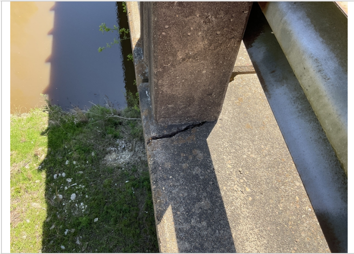
Bridge railing damage RT side
