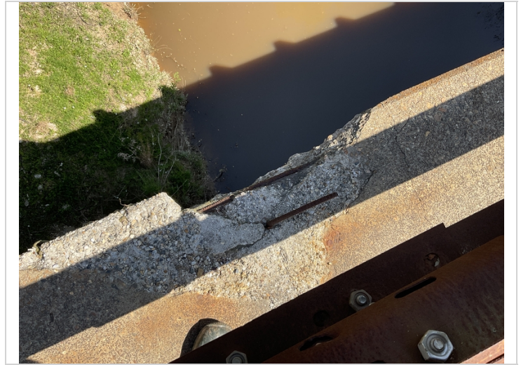
Rebar exposed bridge railing
