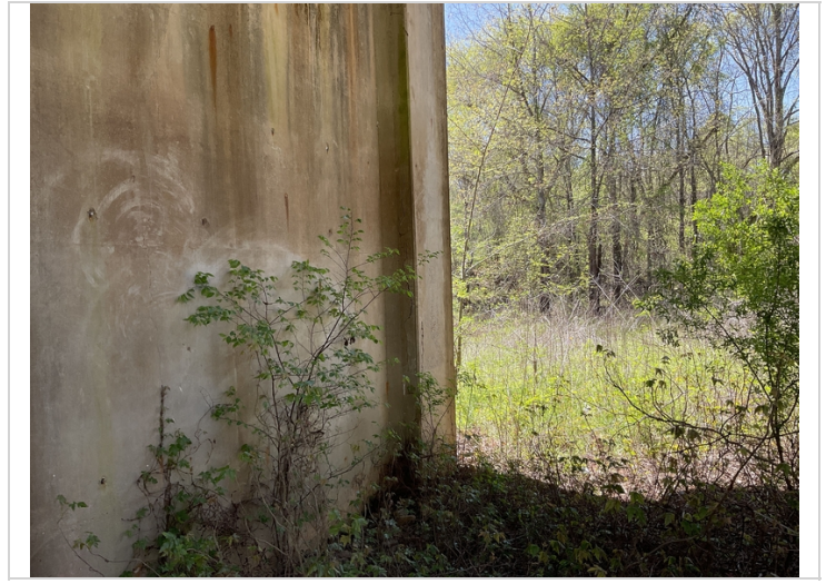
Bent 3 column 1 cracking
